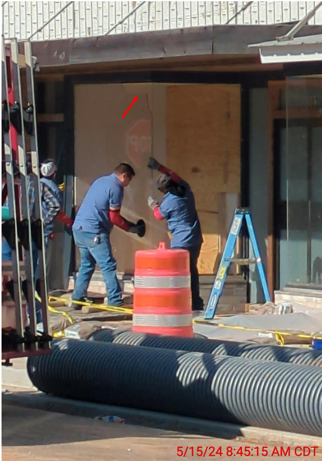
Photo 5: Broken storefront glass (indicated) being removed.
