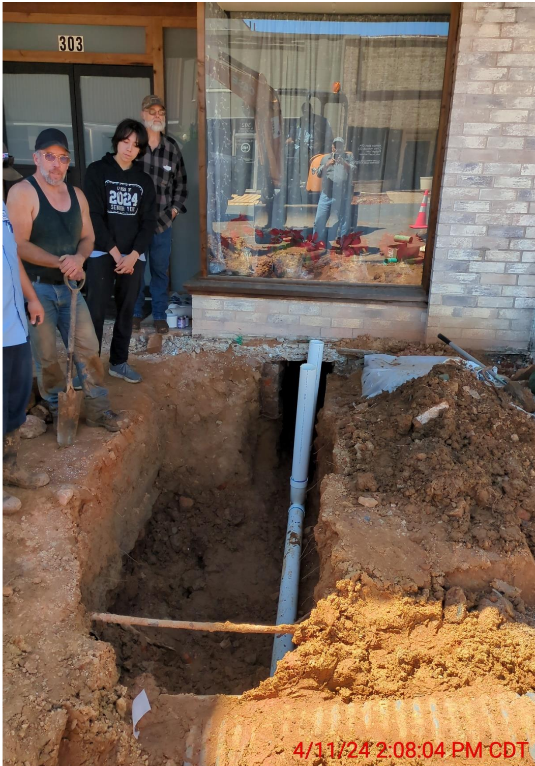
Photo 1: New PVC sanitary sewer line was constructed leading from the crawlspace to the sewer main.
