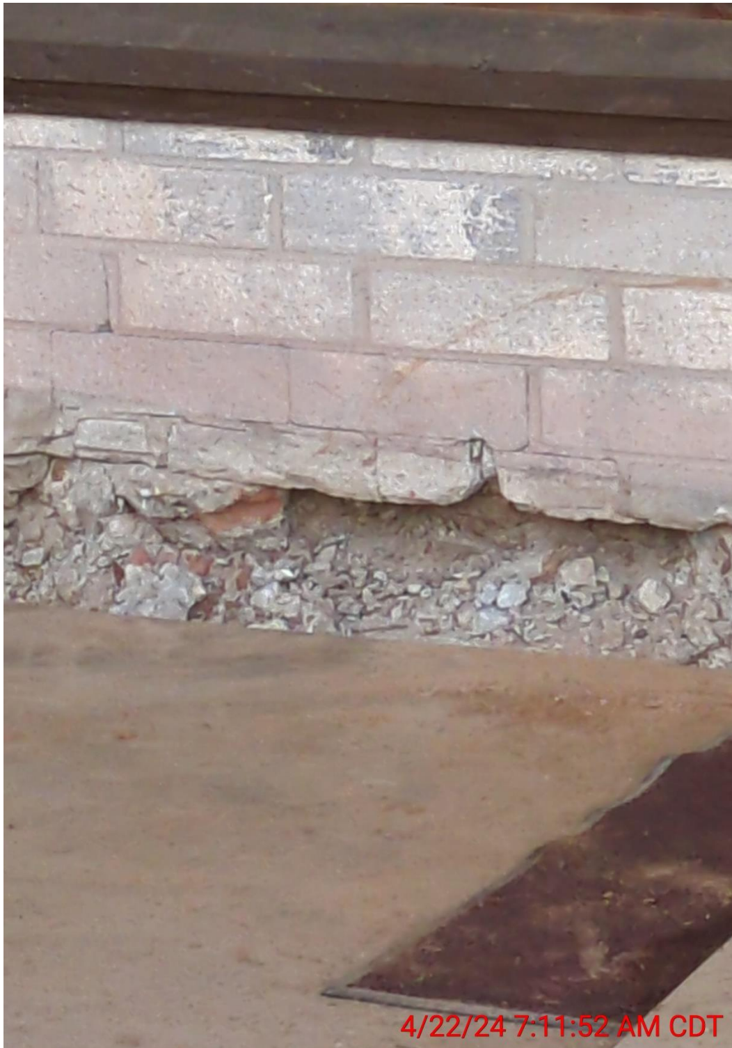
Photo 4: Chip in the brick and a void under the wainscot.
