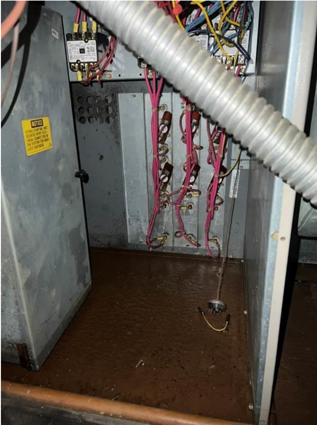
Photo 9: Residual mud in the cabinet of the A/C air handling unit.
