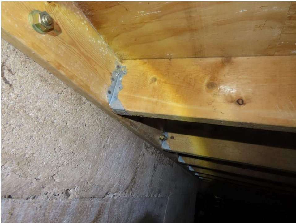
Photo 18: Newer wood framing and metal joist hangers on the ceiling of the crawlspace (the floor framing for the interior above).
