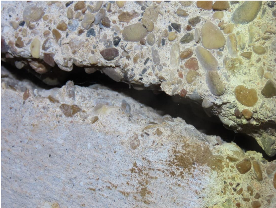
Photo 13: Close-up of the condition depicted in Photo 12 , showing the rounded edges of the fracture.
