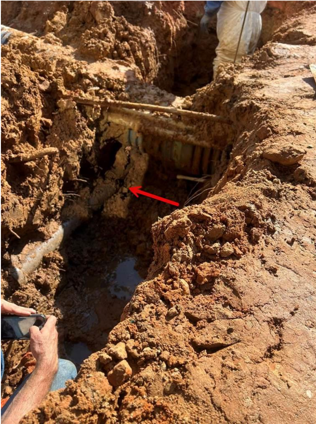
Photo 3: Zoomed out view of Photo 2 showing the position of the break relative to the stormwater pipe.
