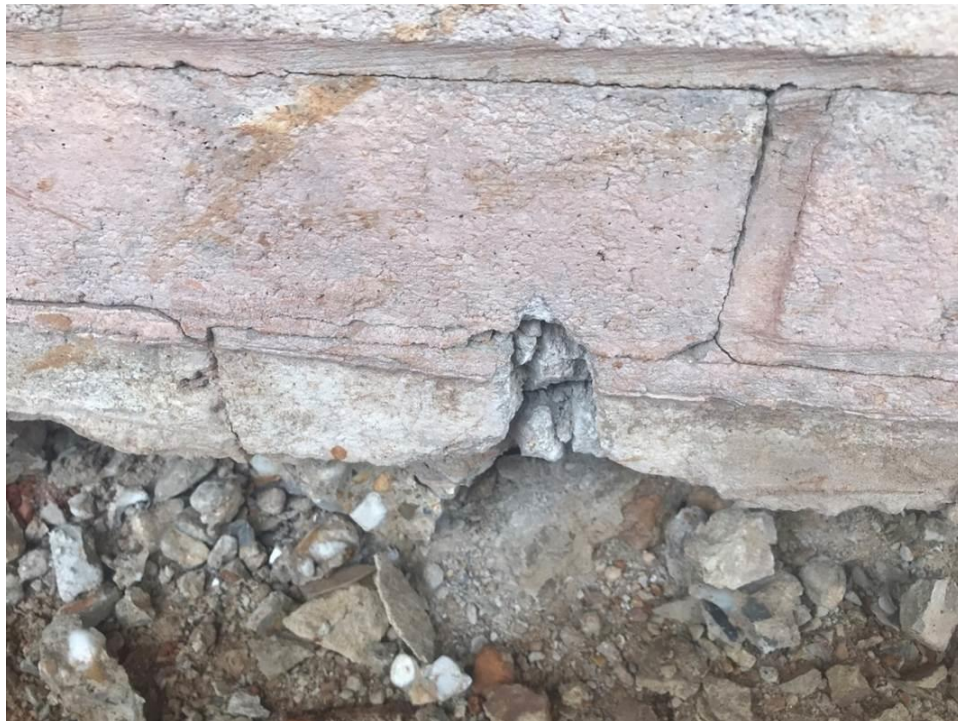
Photo 5: Chip in the brick and a void under the wainscot.
