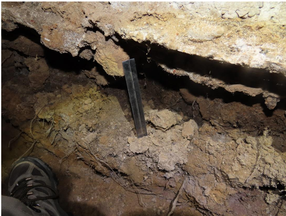
Photo 14: Void in the soil under the beam depicted in Photos 11 through 13 .
