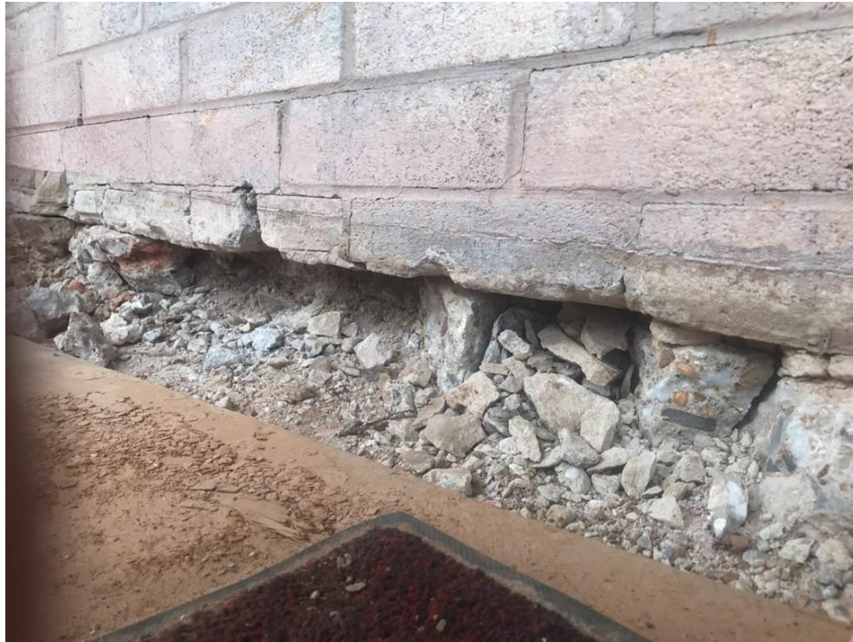
Photo 4: Chip in the brick and a void under the wainscot.
