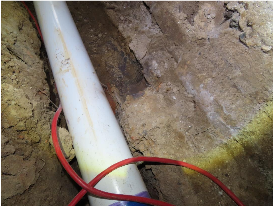
Photo 17: New PVC pipe in the crawlspace.
