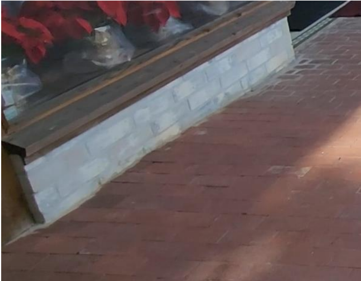
Photo 6: No distress in the brick wainscot prior to construction.
