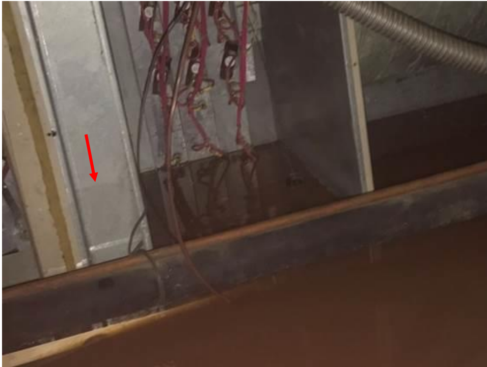
Photo 10: Residual water and mud in the cabinet of the A/C air handling unit. Note the water line (indicated).
