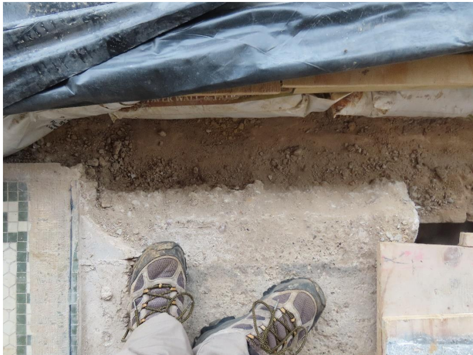
Photo 8: View showing the distinction between the sidewalk base and the top of the grade beam.
