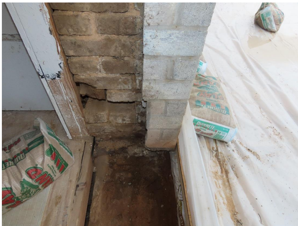
Photo 6: The structural brick was directly supported by the grade beam, but there was a several-inch-tall gap between the top of the grade beam and the veneer brick.
